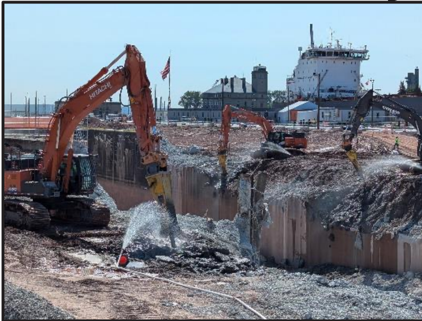
Middle of the Sabin Lock Chamber
