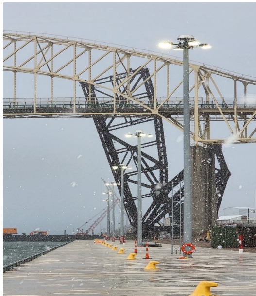
New guard rail, mooring bollards, and LED high mast light poles
