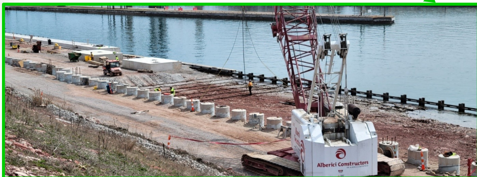
Dead men tie back and mooring bollard foundation installation
