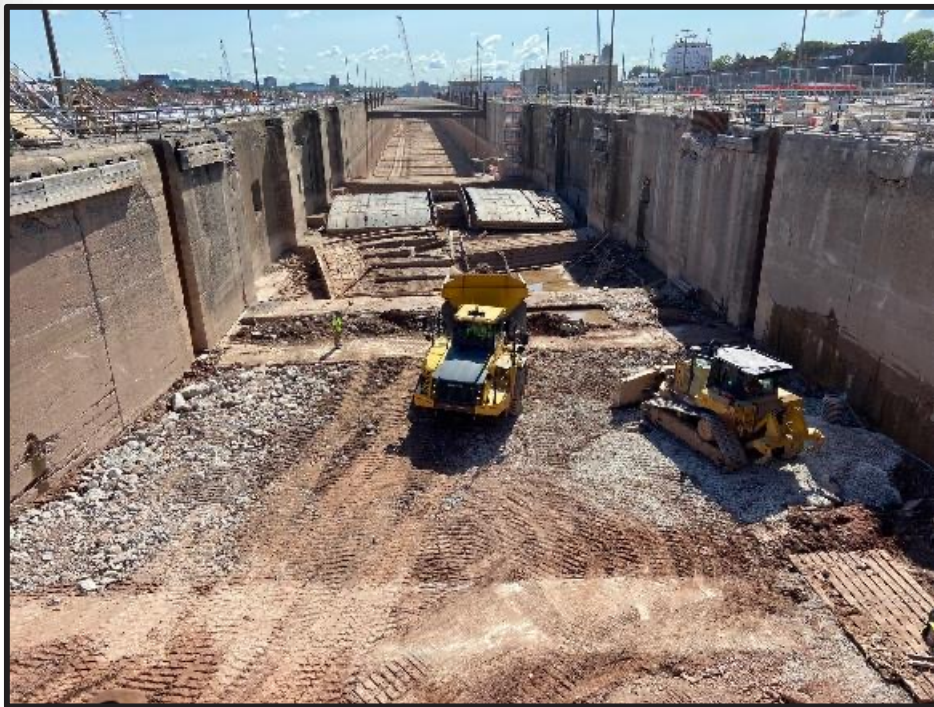
Placement of fill material in Davis Lock
