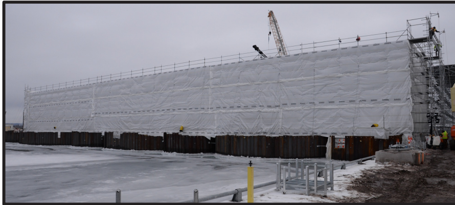
Upstream Cofferdam with Scaffolding Enclosure
