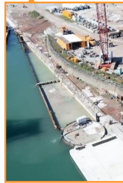
SSP Transition Wall: Tremie concrete placement behind SSP wall face
