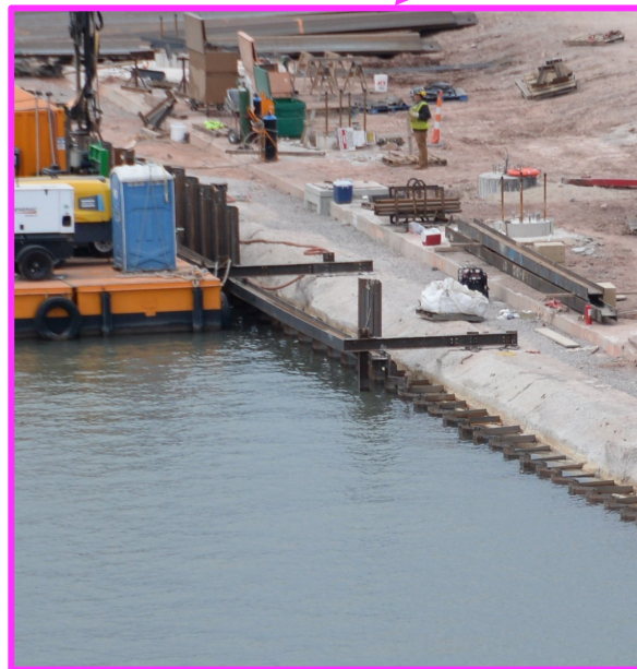
SSP Face Wall: Placement of steel sheet piles
