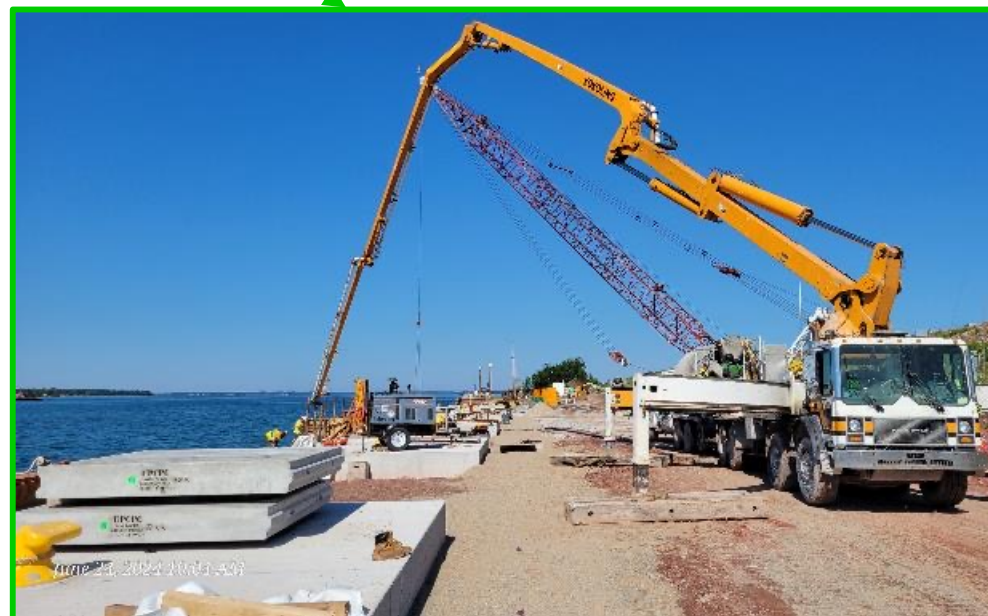
Placement of tremie concrete behind concrete panels
