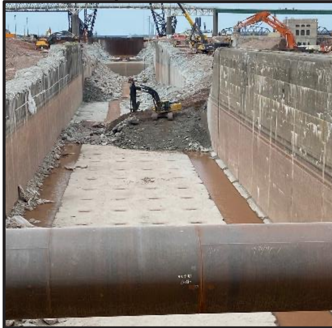
Ramp through North Sabin Lock wall to Sabin Lock floor
