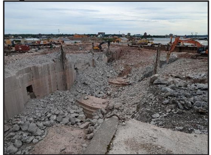
Downstream end the Sabin Lock Chamber
