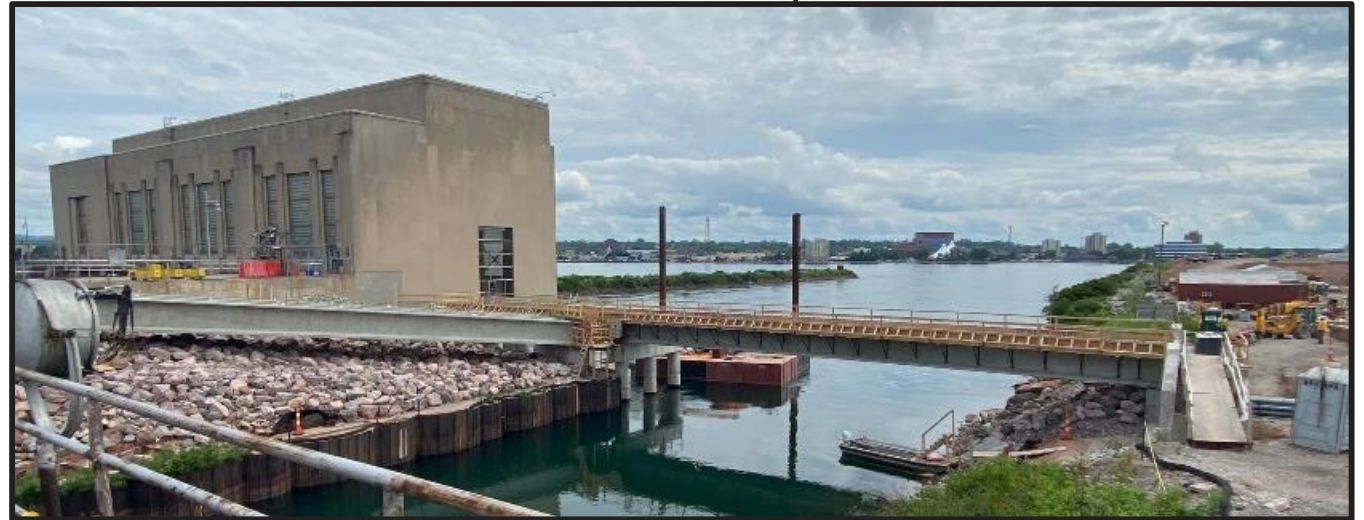
New bridge to the hydropower plant
