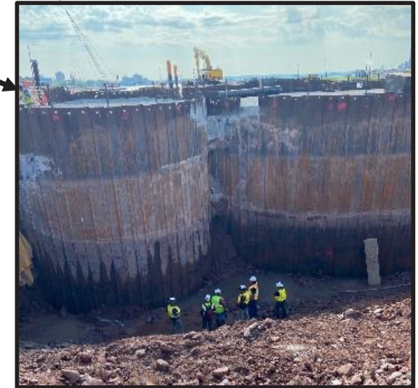
USACE inspection of the Downstream Cofferdam
