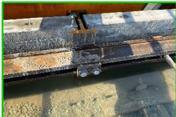
H-Pile, concrete panel, water, and tie rod
