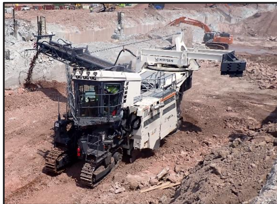
Wirtgen milling machine to be used for bedrock excavation
