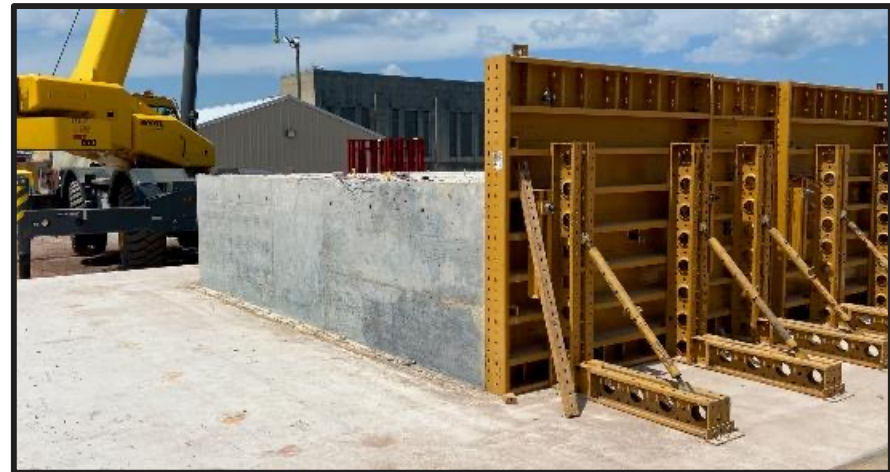
Mass concrete test section
